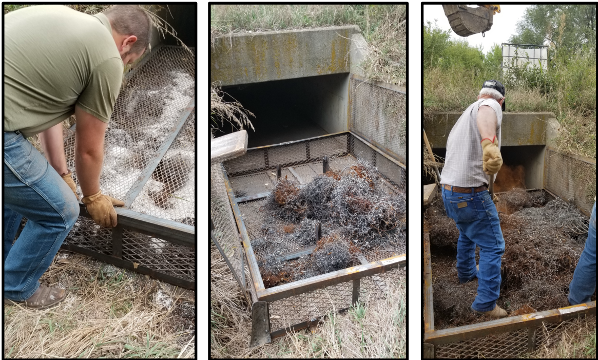
Figure 15. Phos Box installed above the Marion Reservoir/Lake
