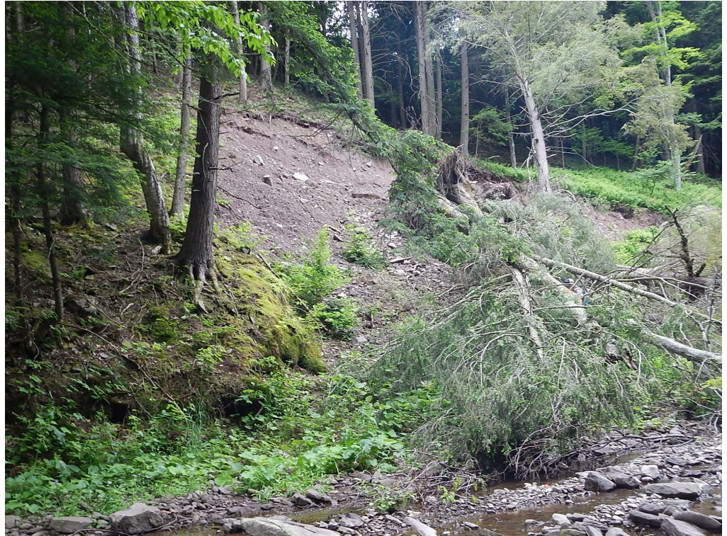
Before the project got started, the stream’s banks were eroding, causing trees and clay sediment to fall into the stream. (Delaware County Soil and Water Conservation District, June 2017)
