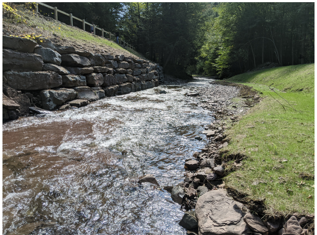
Completed Project. (Delaware County Soil and Water Conservation District, Nov. 2021)
