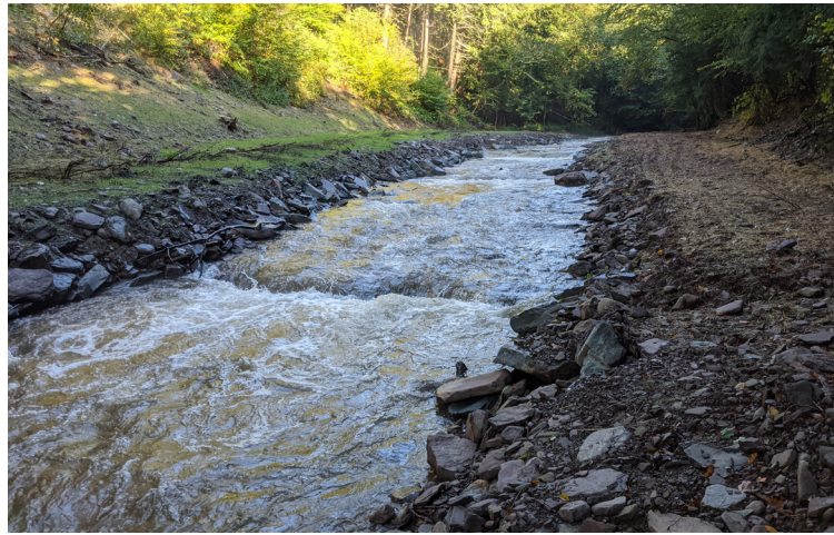
Completed Project. (Delaware County Soil and Water Conservation District, Nov. 2021)
